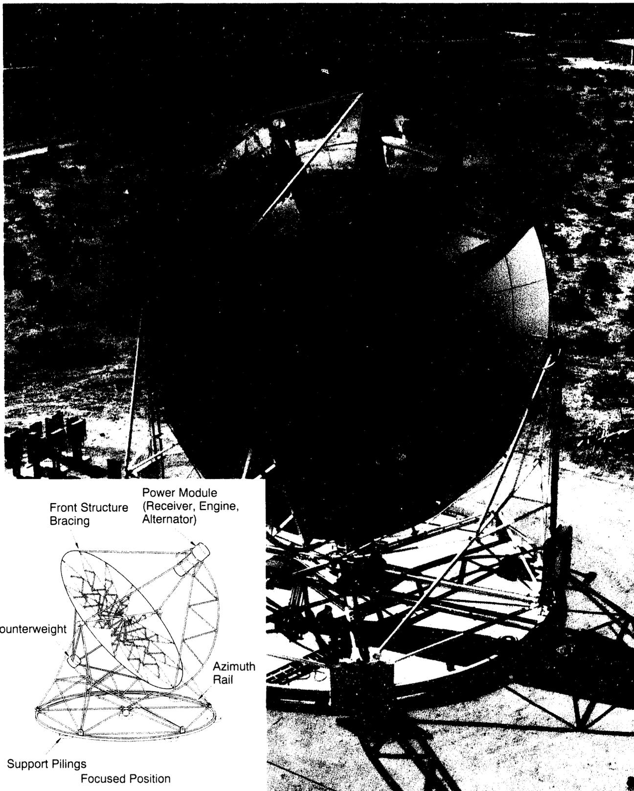
Figure 5-4. General Electric PDC-1 concentrator.
